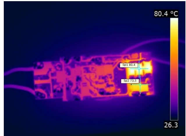
Figure 28 – Bottom Side. R12- Passive Bleeder Resistor: 80.4 °C.
